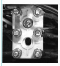
If 120v is demanded, included with this manual is an accessory packet that is needed to change the motor to 120v. Please note the added bridge setup for 120v operation as pictured below and detailed in the wiring diagram.
